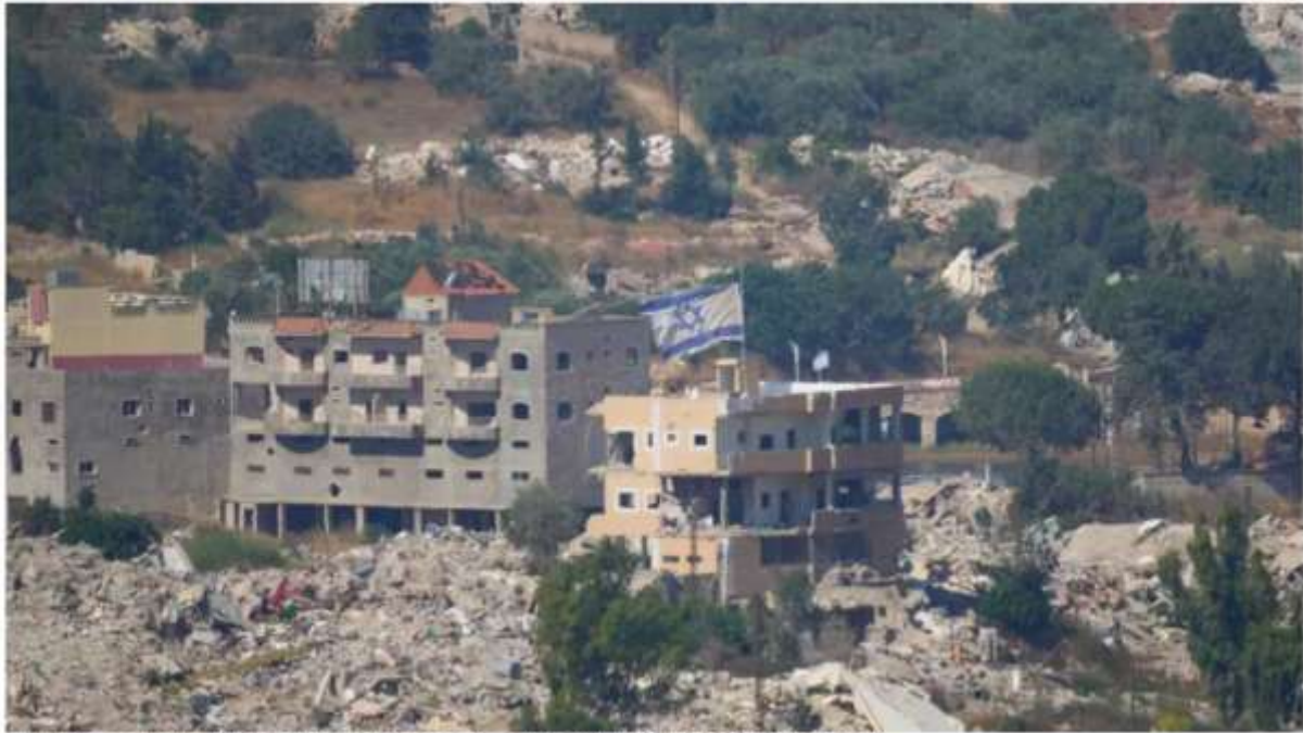
An Israeli flag tops a destroyed building in southern Lebanon, as seen from northern Israel, June 28, 2026. © Ohad Zwigenberg, AP
